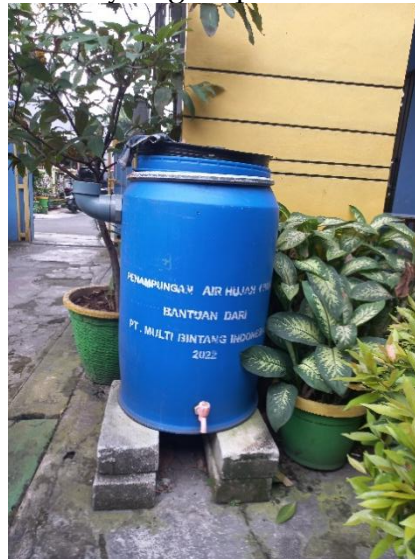
Photo 3. Flamboyan group rainwater harvesting
